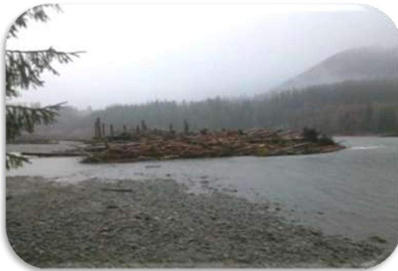
Figure 9. Engineered logjam with racked wood debris.
