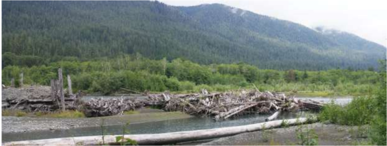
Figure 36. ELJ placed by QIN during the 2008 pilot project (left), accumulating decked wood from river contributions (right). Main channel is in background, and new side channel is forming in foreground.
