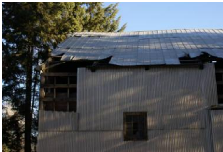
Figure LXXXVIII. Example of windstorm damages to a structure near Rocky Point, on State Highway 5, west of St. Maries.
