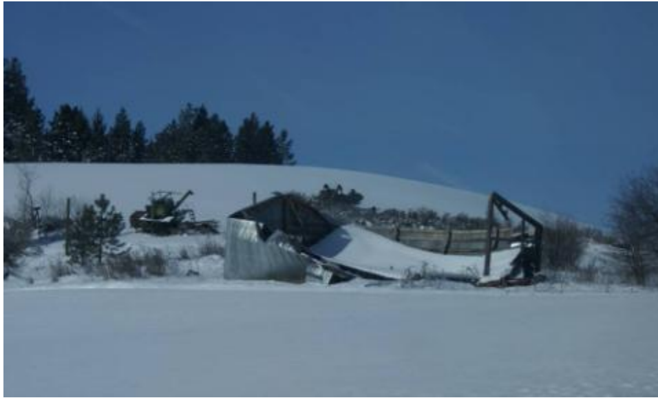
Figure XXXIX. Structural collapse under snow load along US 95, south of DeSmet and north of Sanders in February 2009.
