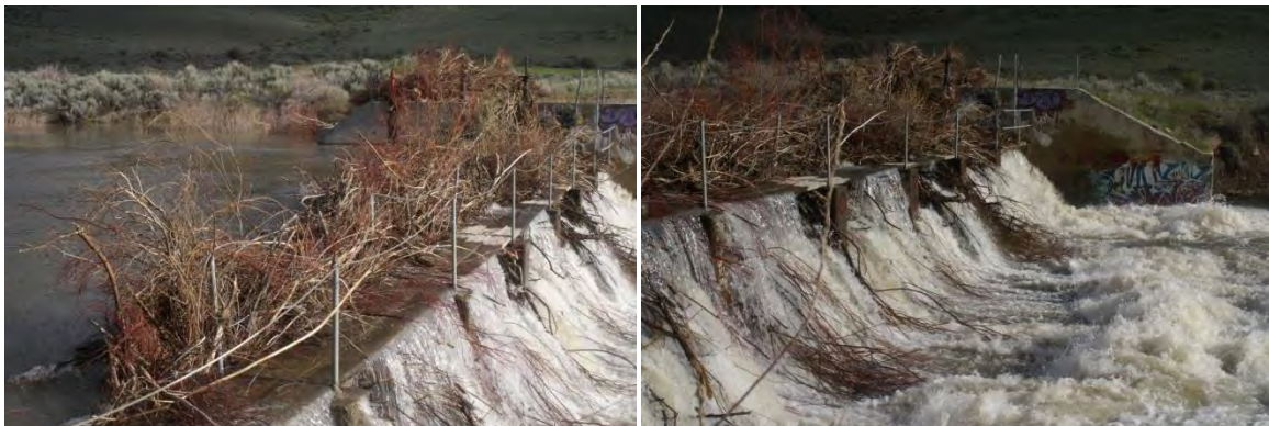
Figure 66. May 19, 2011, debris flow over the China Town Diversion Dam
