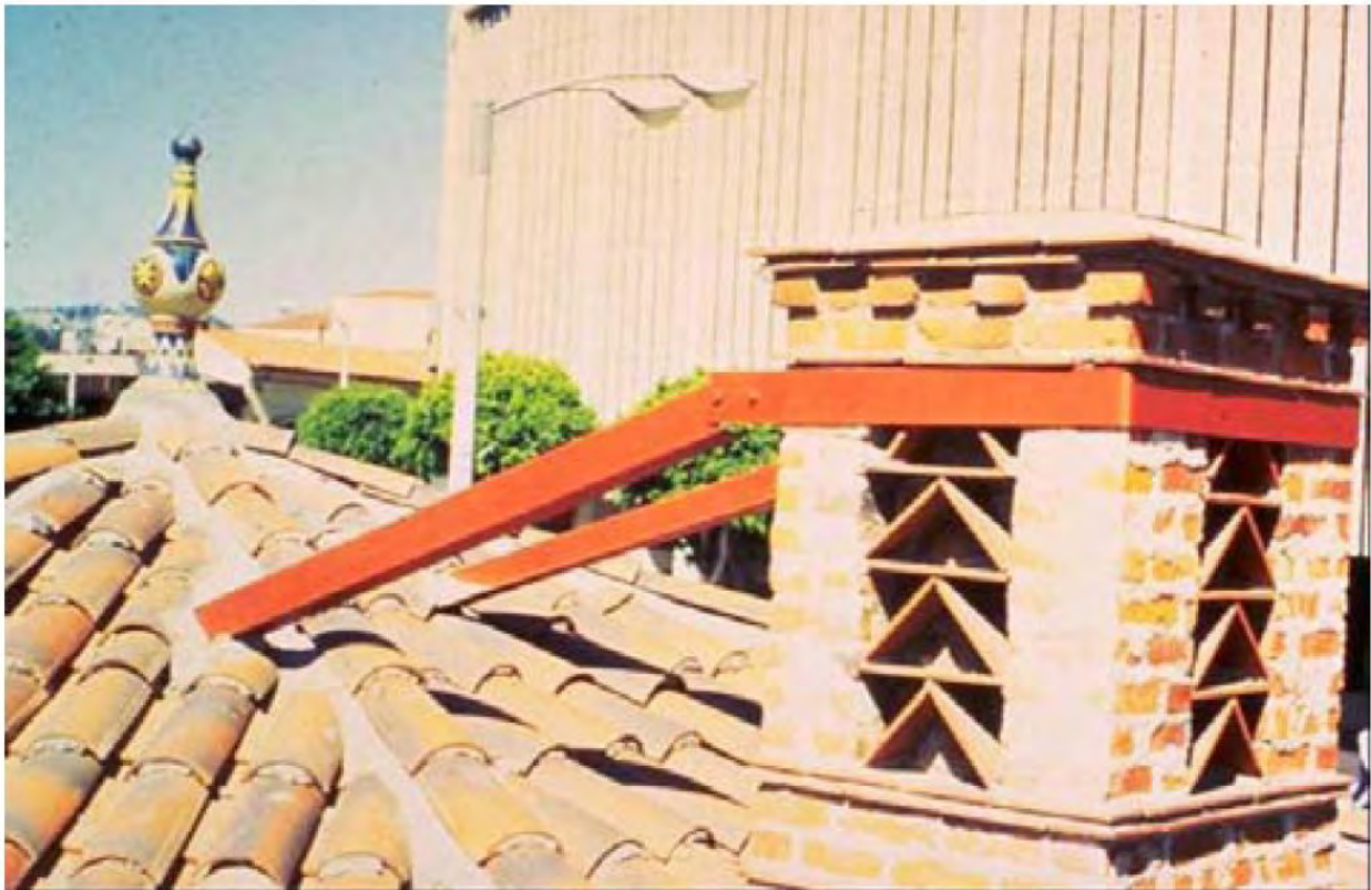
Figure 97. The reinforcement of URM chimney structure (FEMA 2011).
