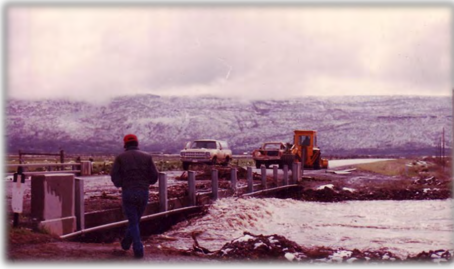
Figure 45. 5/15/1984, National Guard Bridge, Owyhee River. Approach was cut on near side to relieve water flow pressures.
