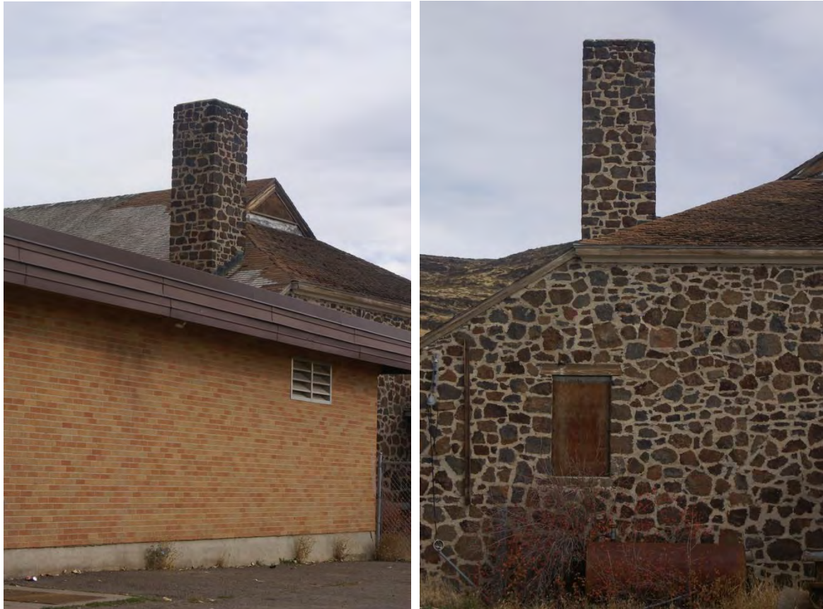
Figure 90. (Left) Unreinforced masonry building in background, with new masonry construction in the foreground. (Right) slate rock with low-strength lime mortar – building currently vacant.
