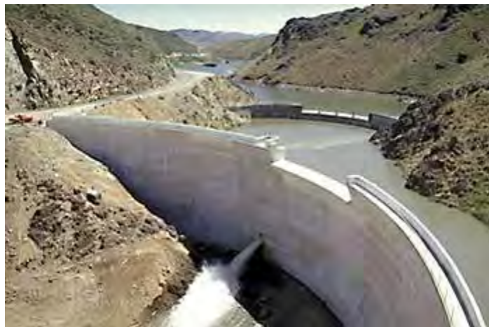
Figure 71. Wild Horse Dam on the Owyhee River showing first dam and replacement dam.
