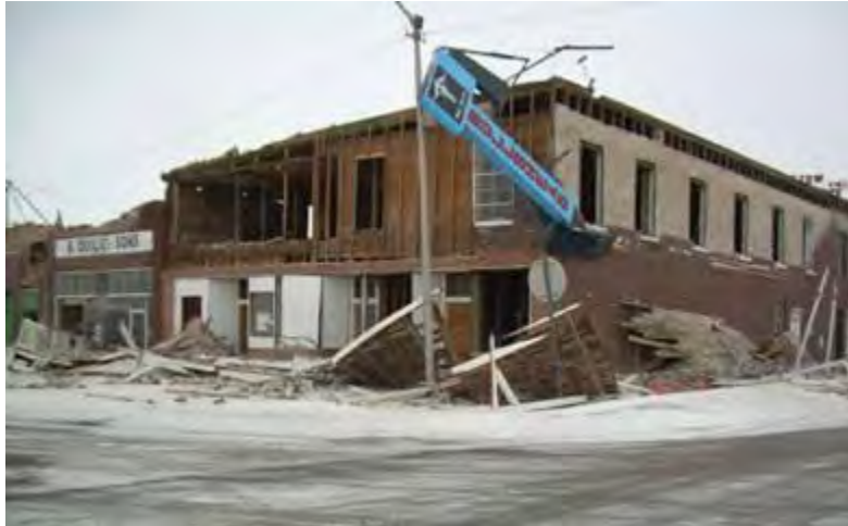
Figure 84. Unreinforced masonry building in Wells, Nevada after M8.0 earthquake in 2008.
