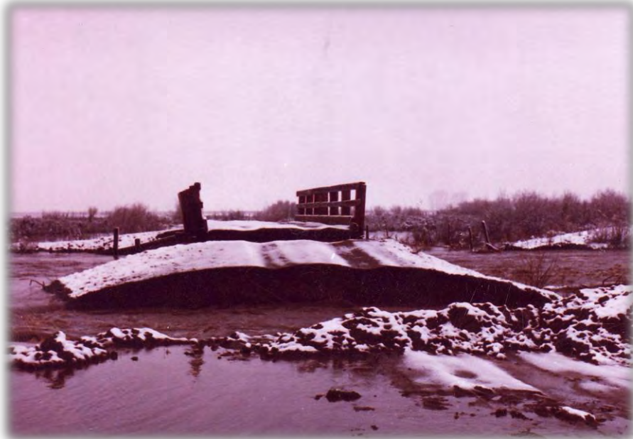
Figure 45. 5/15/1984, National Guard Bridge, Owyhee River. Approach was cut on near side to relieve water flow pressures.
