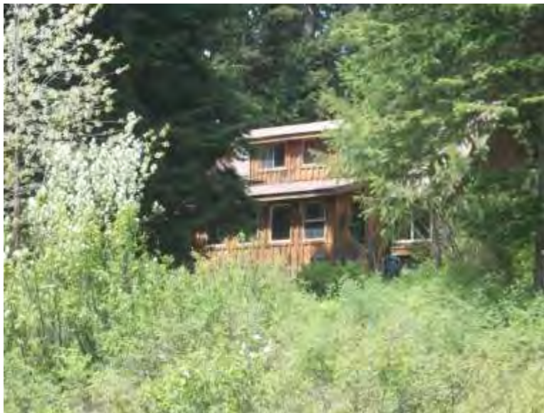
Figure 68. Combustible wood siding structure with heavy wildland fuels abutting.
