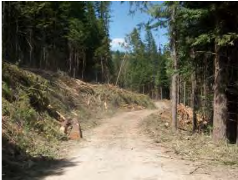
Figure 152. St. Maries River Road improvements between St. Maries and Alder Creek.
