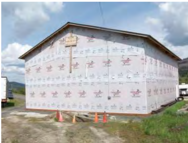
Figure 74. On-going construction to new Emida Fire Department.
