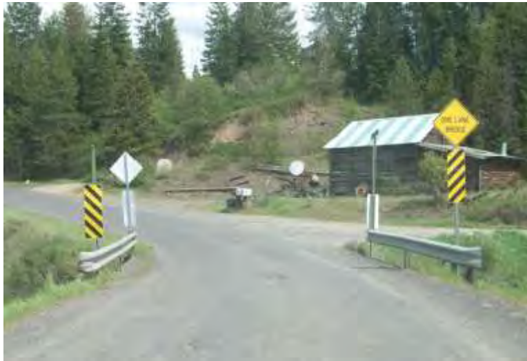
Figure 73. One lane bridge, needing weight-limits posting.
