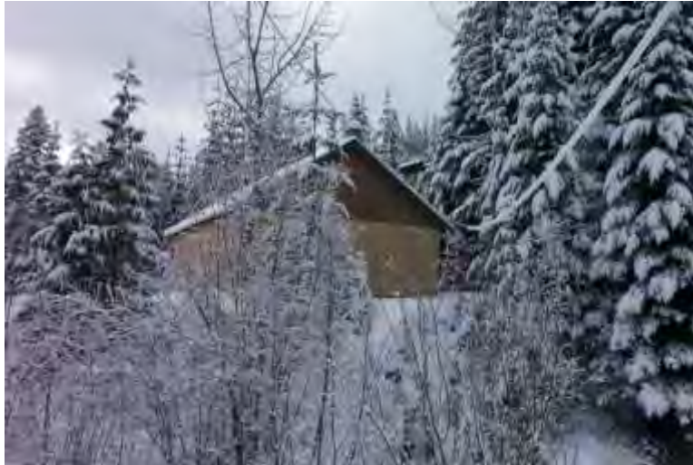
Figure 178. Wildland fuels build-up adjacent to home with power line through trees.
