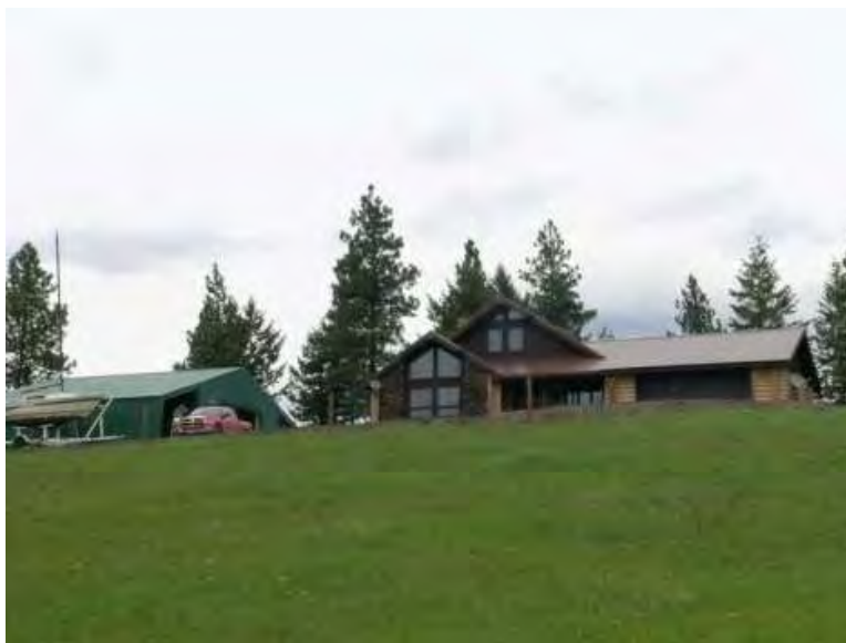
Figure 157. Good defensible space surrounding structure in town.
