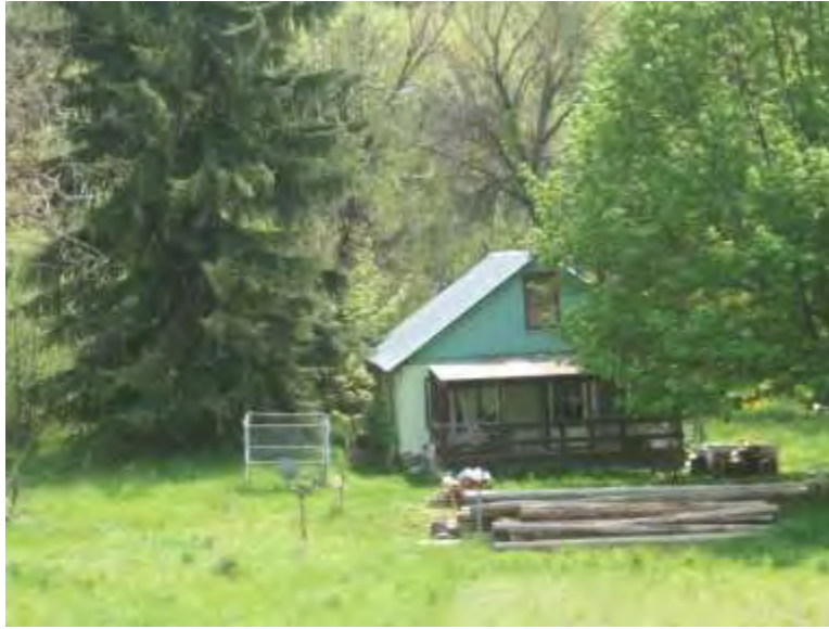
Figure 137. Wood siding home with wooden deck; excess fuels surrounding home.
