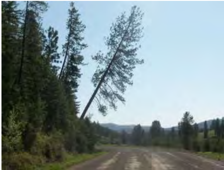
Figure 42. Trees overhanging roads need to be cleared for safe passage.
