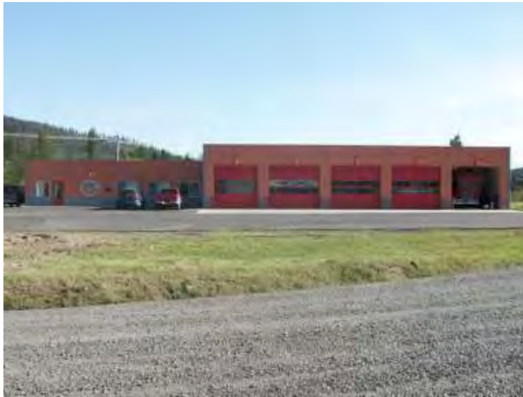
Figure 122. Gateway Fire Department located in Plummer, Idaho.
