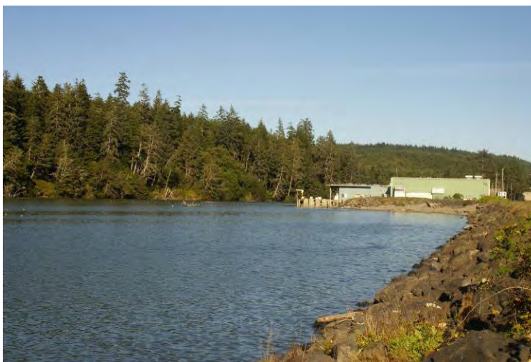
Figure XXXVIII. The Quinault River retaining wall at Taholah.
