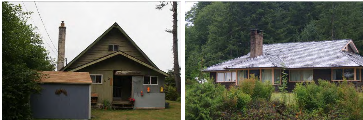
Figure LXVI. Examples of URM Chimney Structures on the QIR, Point Grenville (left) and Amanda Park (right).
