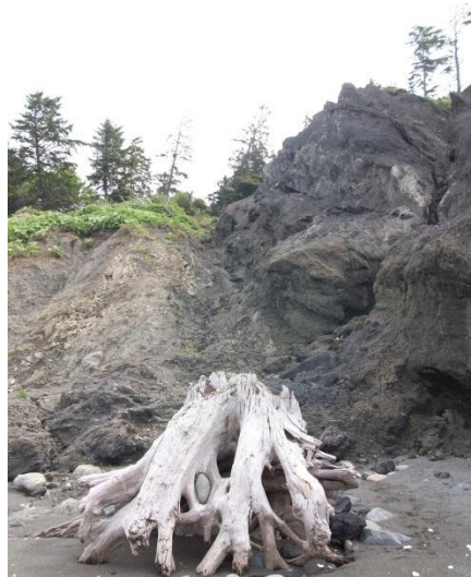
Figure 43. Fault line separating the northern edge of the Duck Creek Diapir (right) and the Quinault Formation (left).
