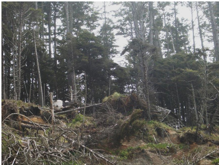
Figure 10. Failed cabin along the shoreline cliff located north of Tunnel Island.
