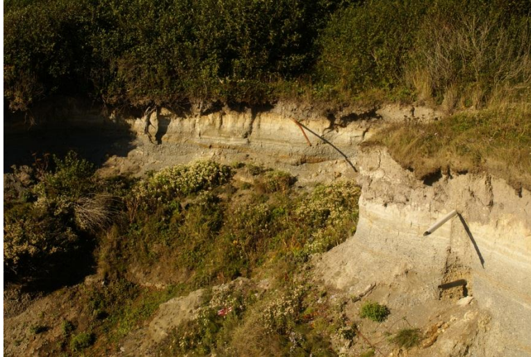
Figure 13. Eocene Sedimentary Rocks of Point Grenville where the US Coast Guard Station water lines are now exposed to show where they once were buried underground.
