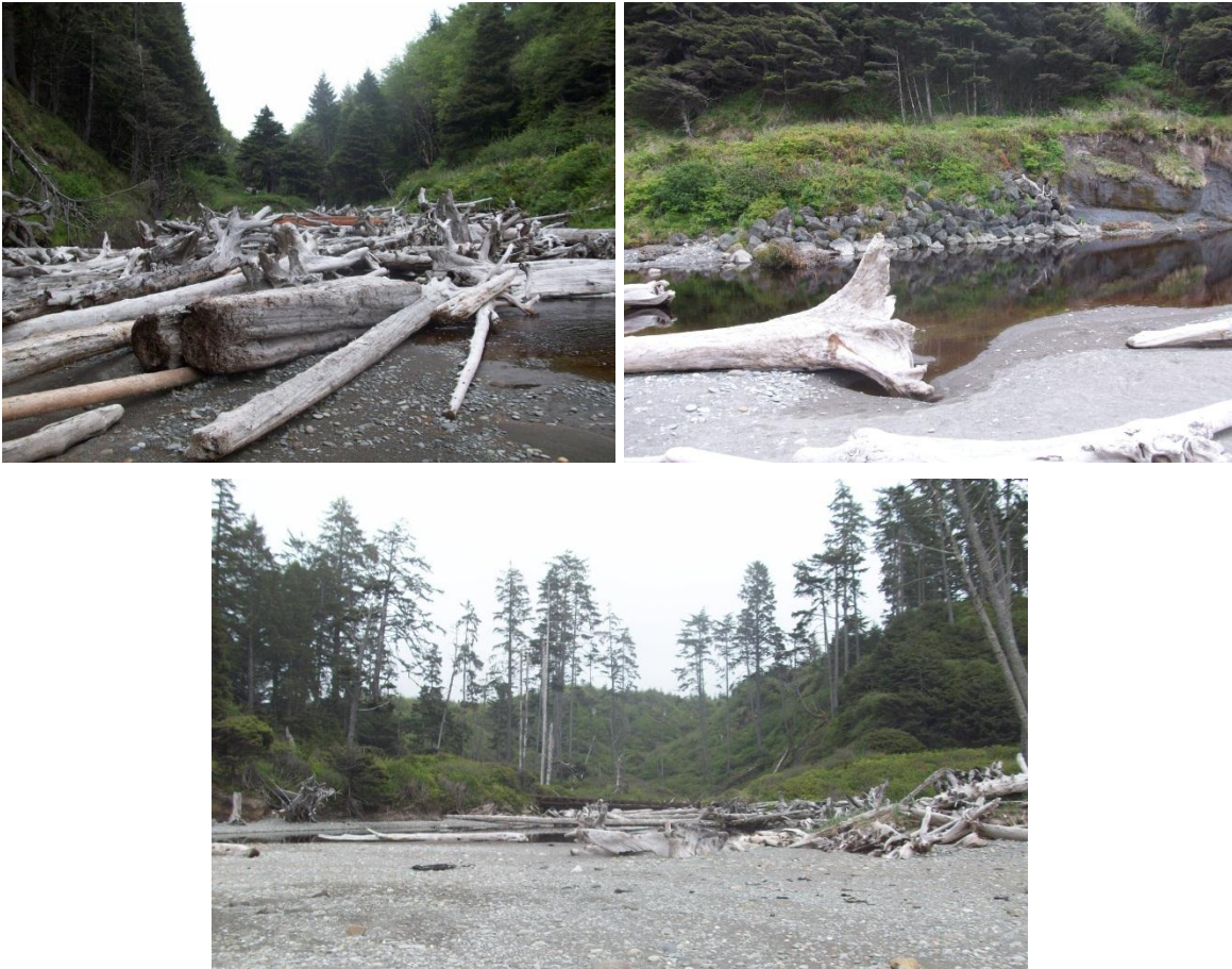
Figure 65. North Fork Whale Creek (left) notice bridge remnants upstream colored red, and rip-rap placed along the road bank between the Whale Creek forks (right), and the South Fork Whale Creek bridge (lower).
