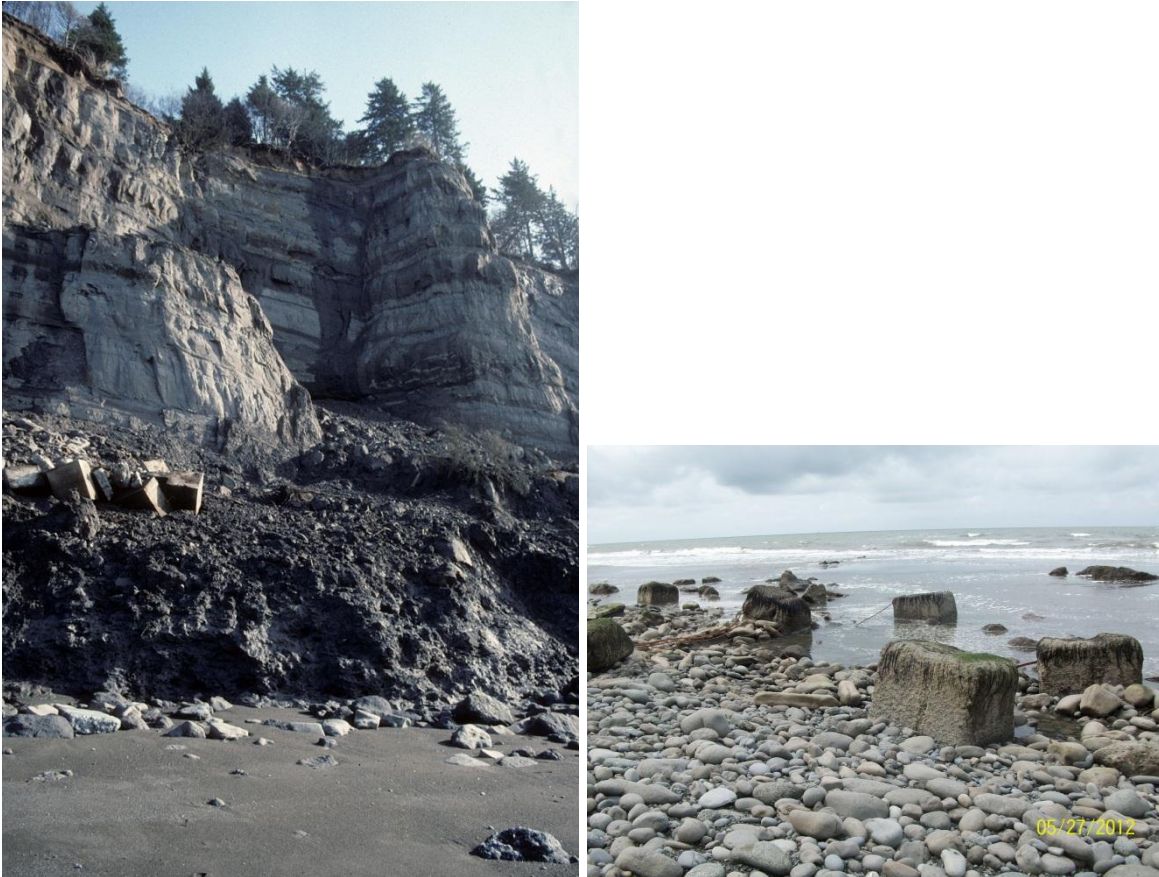
Figure 41. Concrete foundations from the WWII Artillery Bunker Site north of Cape Elizabeth, avulsed to the ocean shorelines from 210' above. Left photograph February 1993 (Workman 2012), right photograph May 2012.
