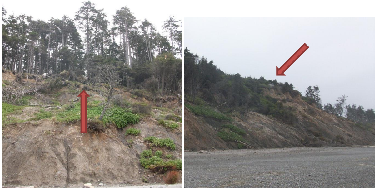
Figure 68. Cliff crest avulsion along the sand and conglomerate cliff tops near Whale Creek that have compromised a cabin (left) and threaten a structure at the crest.
