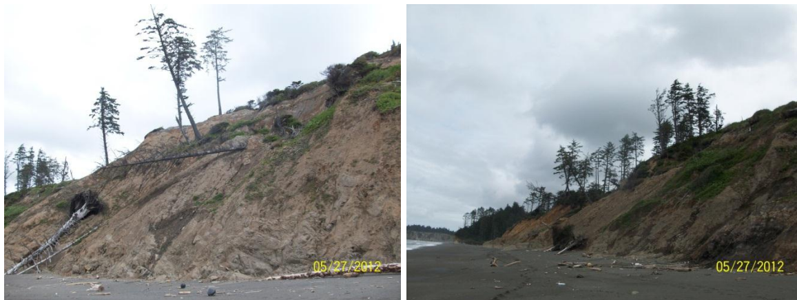
Figure 48. Drunken forests and avulsing wave-cut platform cliff faces in response to destabilized soils near Duck Creek.
