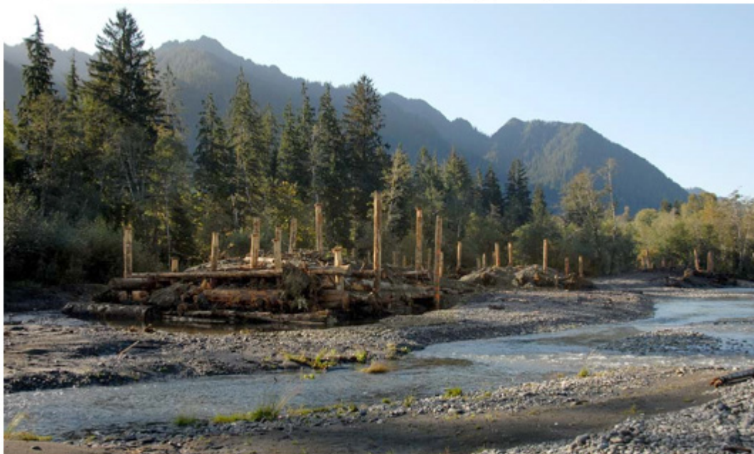
Figure 3: Engineered Log Jams used for salmon habitat loss mitigation [38].
