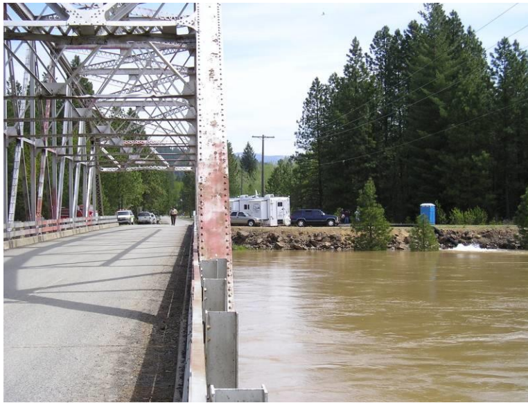
Figure XLII. Bridge approaches were compromised along the Coeur d’Alene River during the May 2008 floods.
