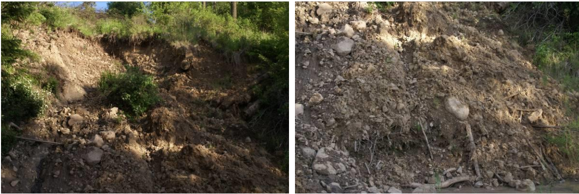
Figure L. Development and construction uphill of this site, caused changes to subsurface water flows, leading to this landslide adjacent to State Hwy 97, near Harrison.
