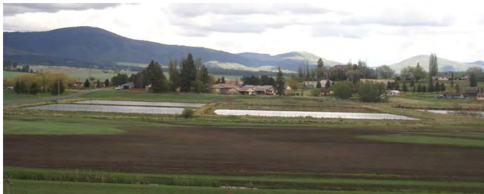
Figure LXVIII. DeSmet Wastewater Treatment Facility (center); farm fields and King Valley drainage in the foreground, the community of DeSmet in the background, and Hangman Creek to the north (left).
