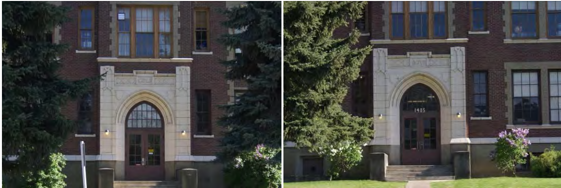
Figure XC. Heyburn Elementary School rests within the Coeur d’Alene Reservation and within the City of St. Maries, and is an example of a high-use URM building.
