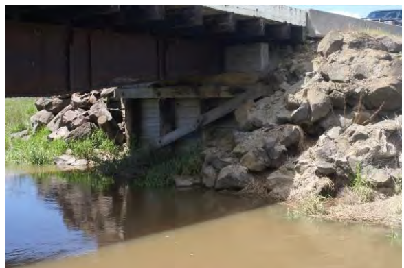
[Above] Local access road crossing Hangman Creek on June 6, 2010, a time of relatively low water flows. The bridge crossing has restricted the width of Hangman Creek and eliminated a major portion of the normally functioning floodplain at this point. The supporting structure of the bridge has been failing and is depositing debris into the river channel.
