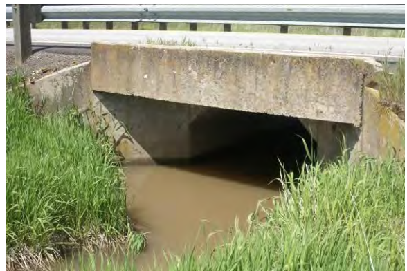
[Above] US95 crossing on June 5, 2010, a time of relatively low water flows. The constriction of the stream for the road crossing causes water to accumulate at the surface upstream of the crossing.
