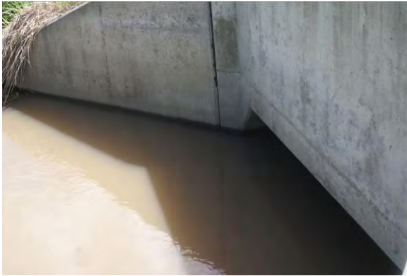
[Above] US95 crossing of Tensed Creek on June 5, 2010, a time of relatively low water flows. Note the absence of freeboard between the water level and the bottom of the road crossing. Both are upstream views.
