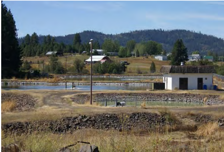
Figure LXXIX. Plummer Wastewater Treatment Facility within the Plummer creek watershed being retired in favor of a new site located above the floodplain.
