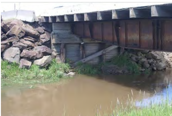
[Above] Local access road crossing Hangman Creek on June 6, 2010, a time of relatively low water flows. The bridge crossing has restricted the width of Hangman Creek and eliminated a major portion of the normally functioning floodplain at this point. The supporting structure of the bridge has been failing and is depositing debris into the river channel.
